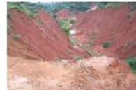
Soil protection, erosion control
